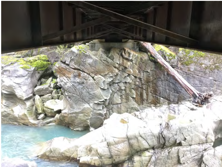
Right Bank Abutment when facing downstream
