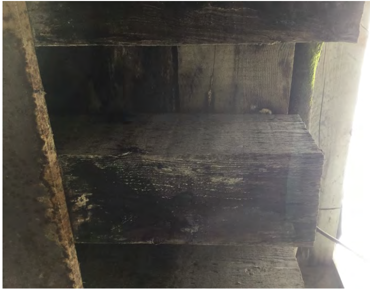
Upstream planks are untreated
