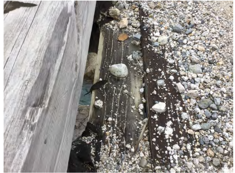
Downstream planks are untreated
