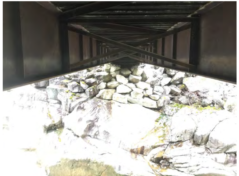
Left Bank Abutment when facing downstream
